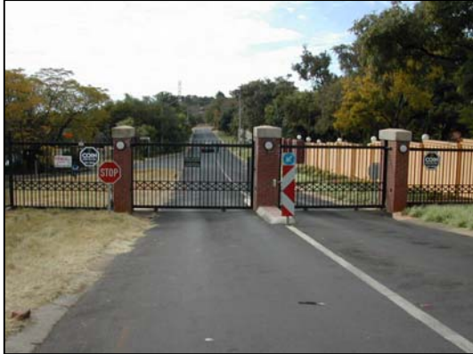
Figure 15: Strubenkop Road entrance
