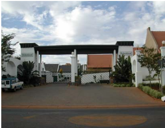
Figure 6: Entrance to large secure townhouse complex in Pretoria
