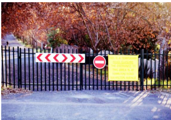
Figure 3: Enclosed neighbourhood in north Johannesburg: road closed through gate.
