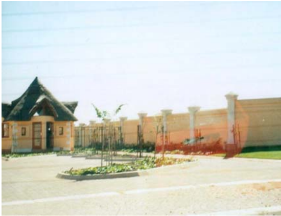
Figure 1: Entrance to large security estate in east Johannesburg
