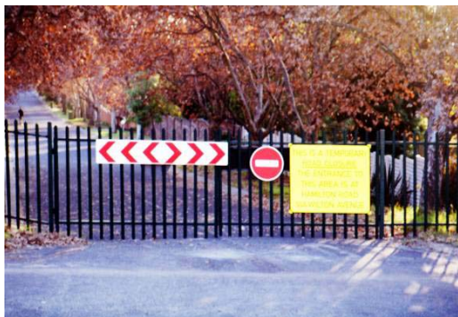
Figure 2: A road closure by means of a palisade gate.
