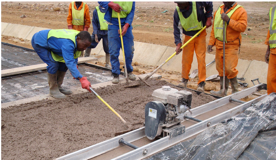
Labour-intensive construction of a low-volume road
