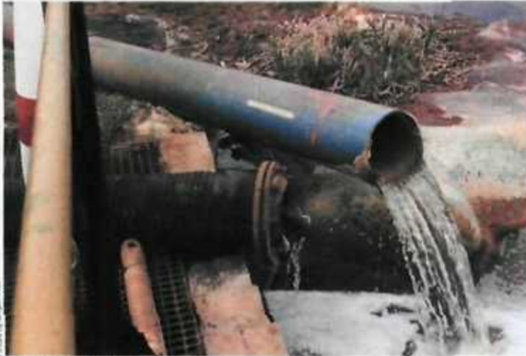
SPILLING OVER Mine water spills into a catchment dam, where it gets treated with caustic soda
