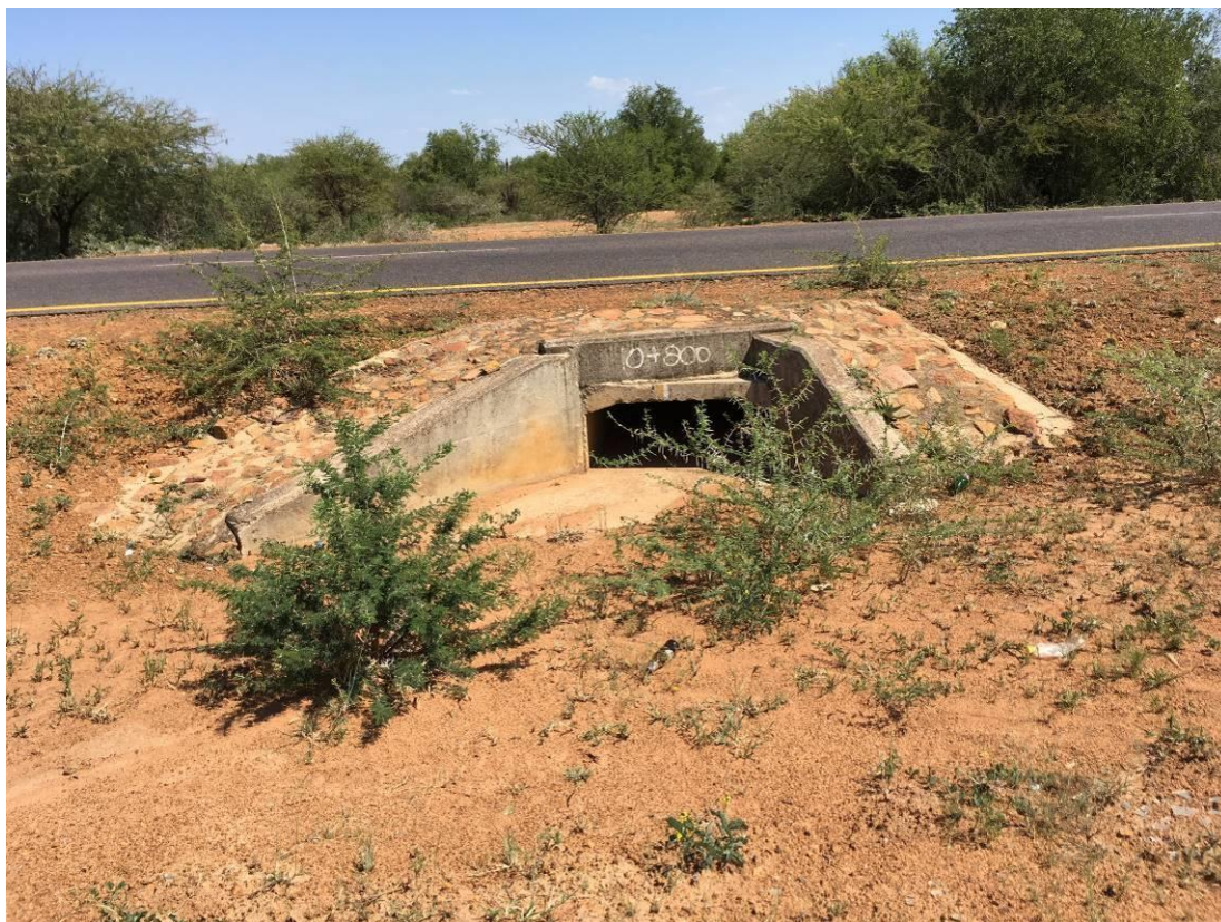
Figure 6.8: The culvert under the road.
