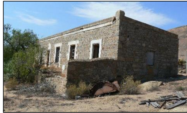
Figure 5-25: Rondekop in the Namaqua National Park has a distinctive stone, flat roofed house with decorative window and door treatment. Source: Webley (2004)
