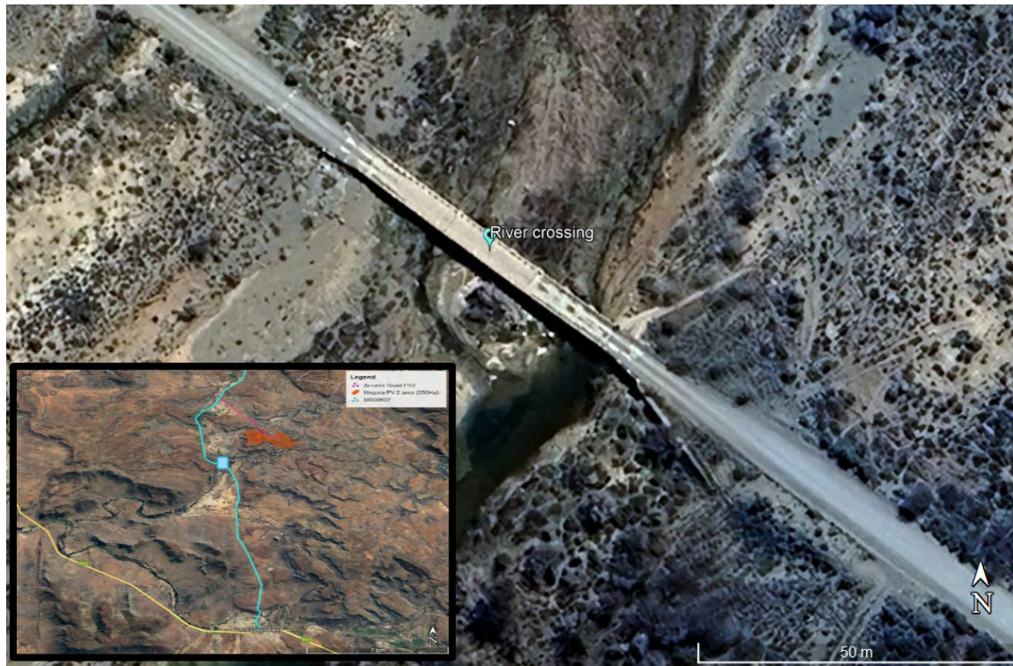
Figure C.3: Aerial View of Bridge located on MR00607 (Source: iWink, 2025)
