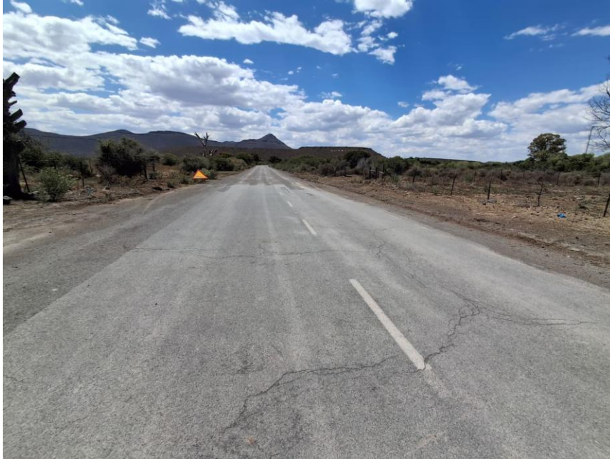
Figure C.2: Start of the MR00607 road in Murraysburg, showing the typical condition of the road (Source: CSIR, 2026)
