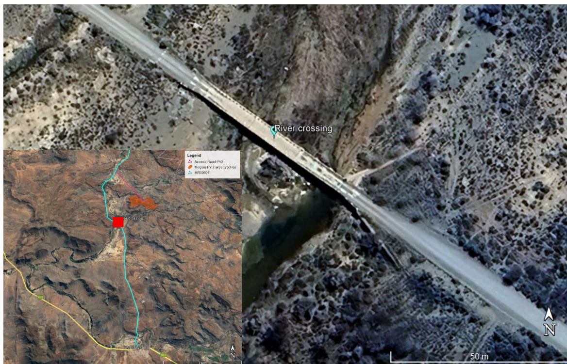
Figure B.6: Aerial View of Bridge located on MR00607 (Source: iWink, 2025)
