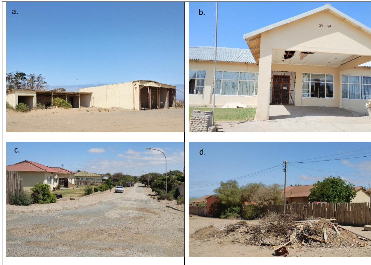
Figure 6-11: Alexander Bay: condition of infrastructure: a) Abandoned buildings, b) Damaged hospital, c) Decaying streets, d) Rubble in streets.
