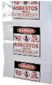
Figure 3: Fragments shall be collected and placed into a suitable container, such as heavy-duty polyethylene plastic bags or steel drums.
