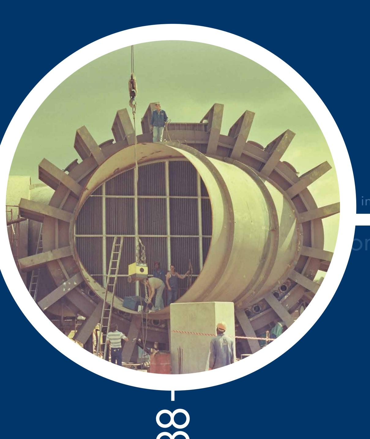
The construction of a medium-speed windtunnel expands the CSIR's aerodynamics research capability. Today, the CSIR's wind tunnels continue to be used in aerodynamic design tests and studies for local and international entities in the aeronautical sector.
