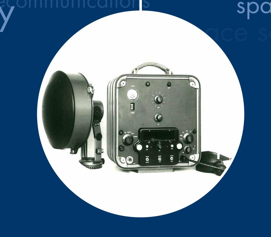
Dr Trevor Lloyd Wadley invents the first microwave electronic distance measurement equipment, the tellurometer. The tellurometer revolutionised land-surveying throughout the world. The company set up to manufacture the tellurometer maintained the market lead for this equipment for over 25 years.
