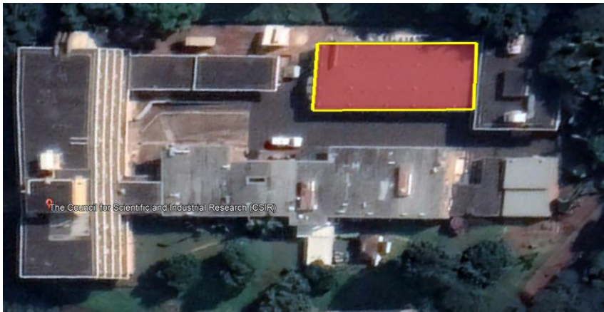
Figure 7-2 Aerial view of the BDF facility
