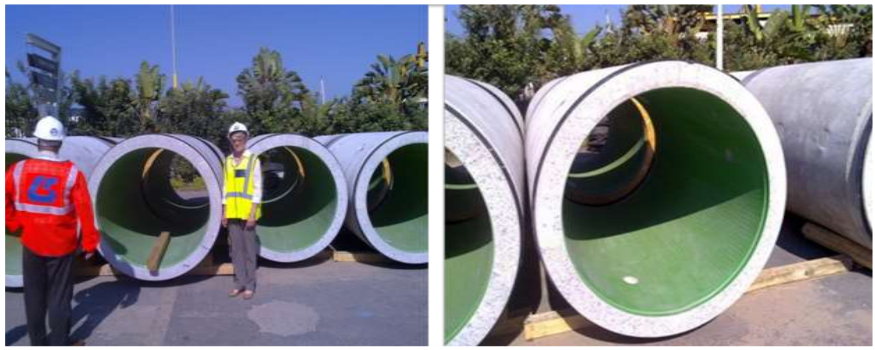
Figure 3-16 Typical Pipe Segments for Jacking at Durban Port Mini-Tunnelling
