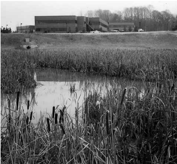
Figure 6.25: Part detention, part retention facility, including an artificial wetland
