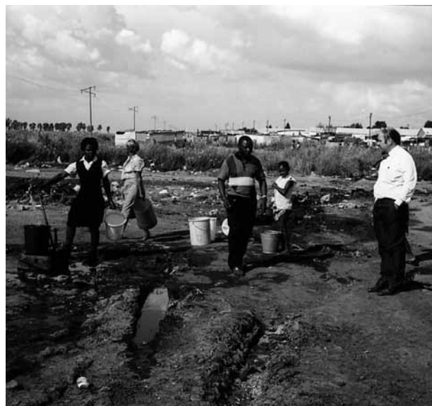
Figure 6.31: This water point has been placed in a low-lying area. Drainage of runoff and water spilled from the point has not been allowed for, and a health hazard has resulted
