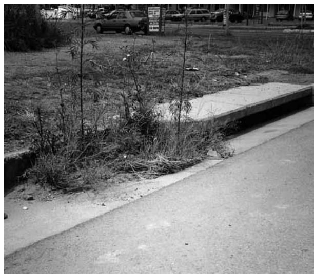
Figure 6.34: Kerb inlets require maintenance
