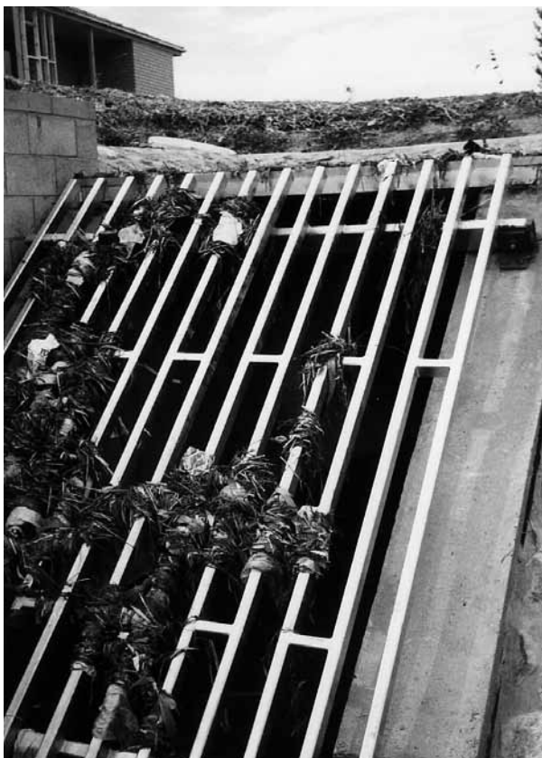
Figure 6.33: Inlet grids need attention
