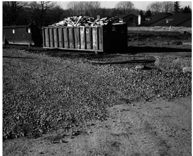
Figure 6.26 (a): Construction sites can be prevented from polluting the surrounding area by the use of straw bales, mulching and geo-mats. Aggregates placed at exits from sites prevent the transport of pollution
