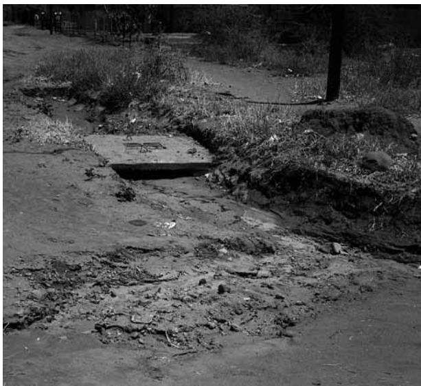
Figure 6.35: The use of underground drainage systems in unpaved roadways should be justified
