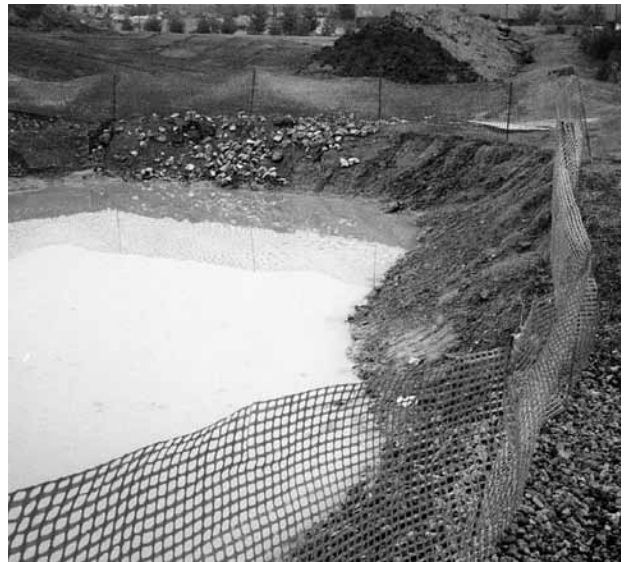
Figure 6.26 (b): Construction sites can be prevented from polluting the surrounding area by the use of straw bales, mulching and geo-mats. Aggregates placed at exits from sites prevent the transport of pollution
