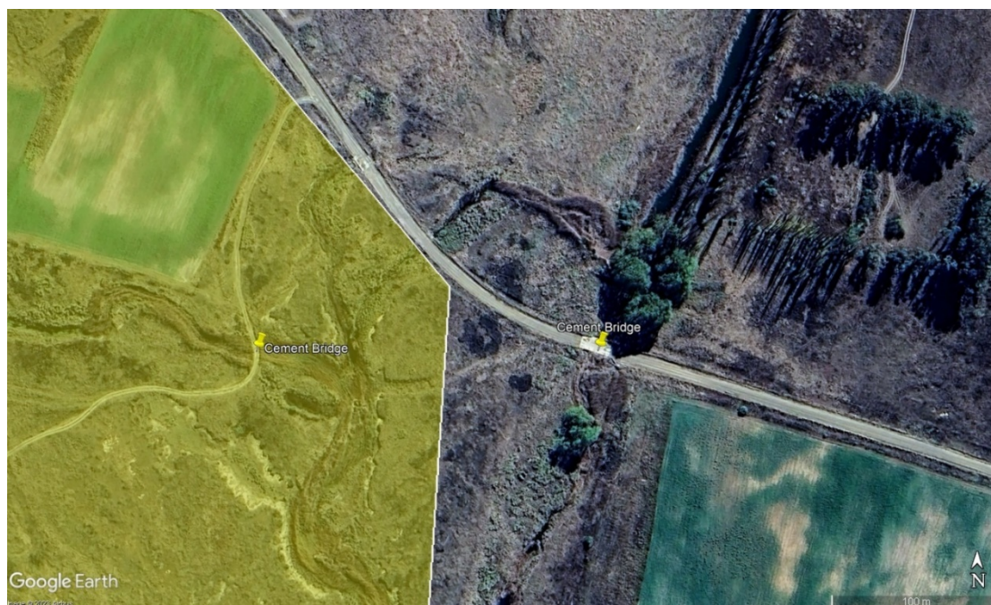
Figure 2.9: Map indicating the relevant cement bridges (Source: Google Earth, 2023).
