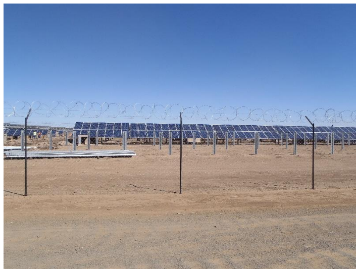
Figure A.7. Example of PV Technology (DEFF, 2019)
