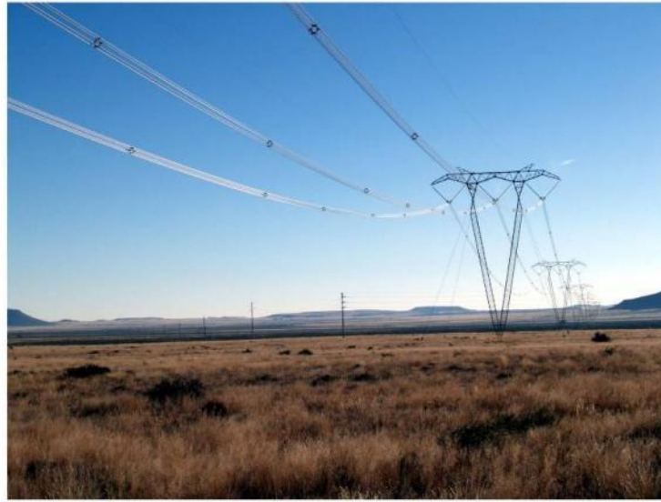
765kV Transmission Pylon @ 250m
