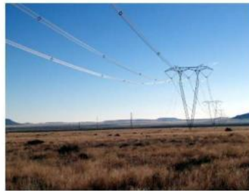
765kV Transmission Pylon @ 500m
