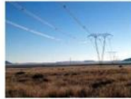
765kV Transmission Pylon @ 1000m
