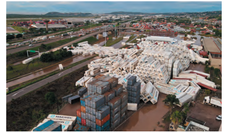
The 2022 floods in KwaZulu-Natal wreaked havoc in the Port of Durban and surrounds.
