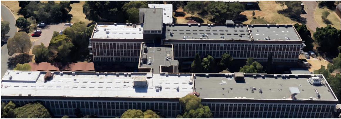
Figure 6 : Building 33 Top view
