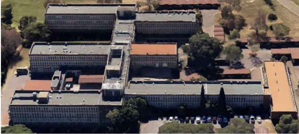
Figure 3 : Building 10 Top view
