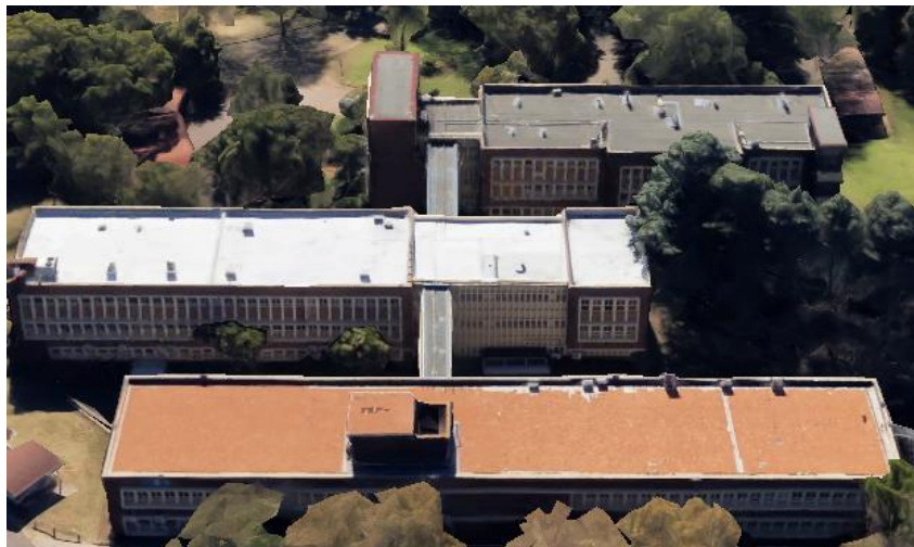
Figure 2: Building 3 Top view
