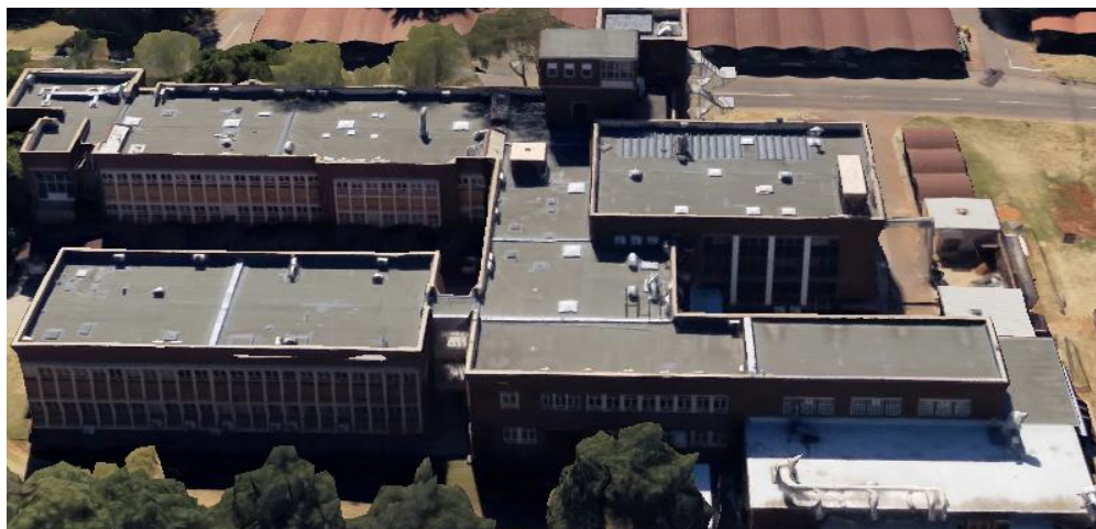
Figure 5: Building 23 Top view
