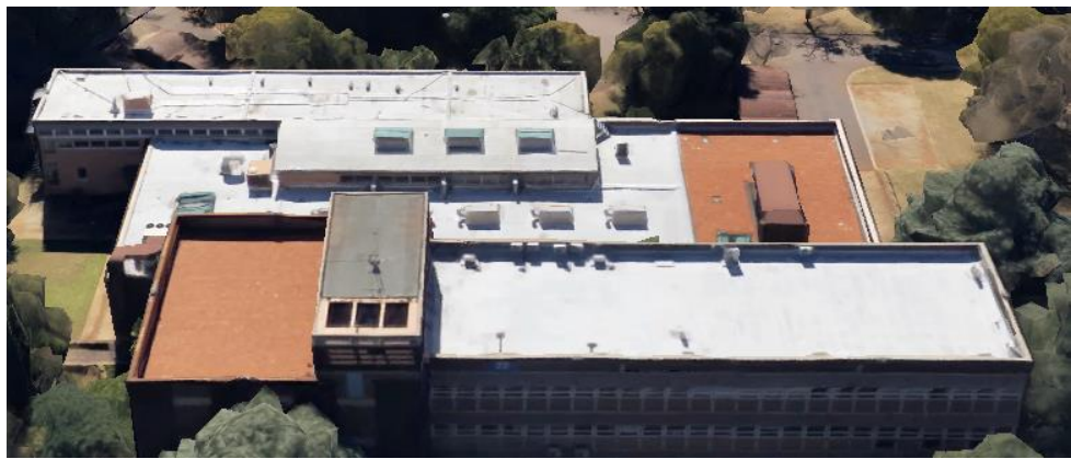
Figure 4 : Building 22 Top view
