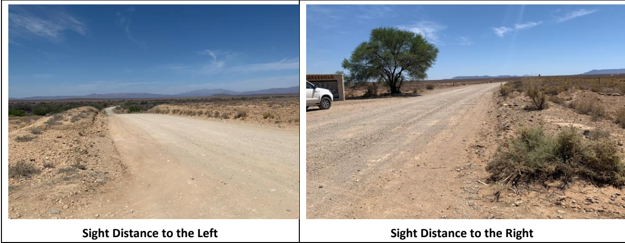
Figure 9: Sight Distance at Existing Access at Km 74.84 along MR319
