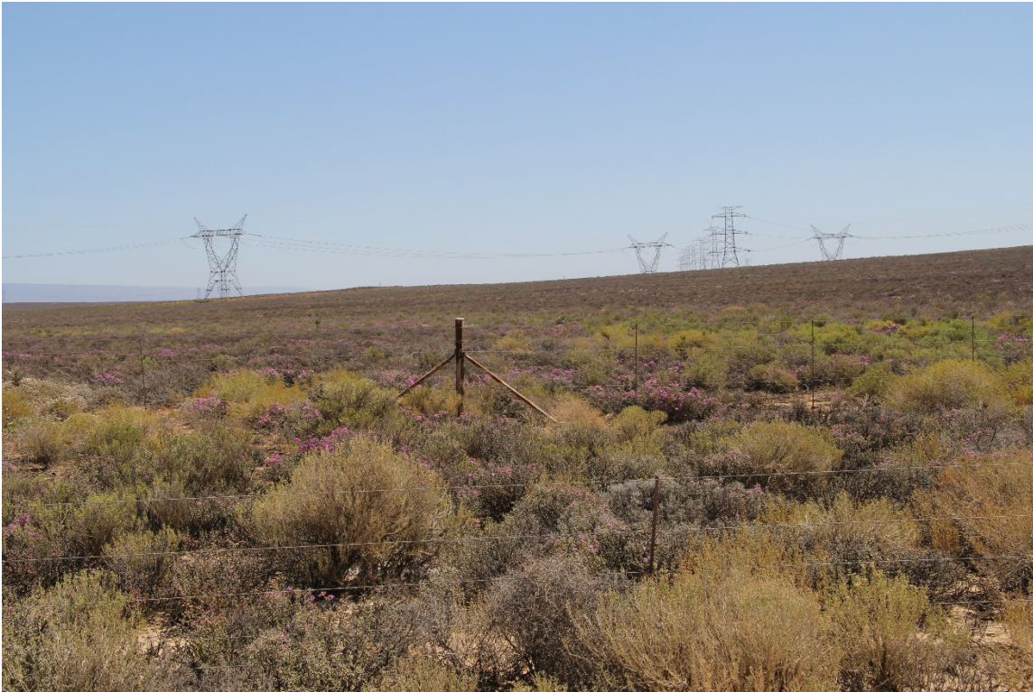
Figure 15: View of existing power lines on Die Brak Farm (Photo: L. Kellerman)
