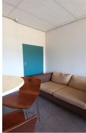
Furniture to be removed, tiles, ceiling replaced
