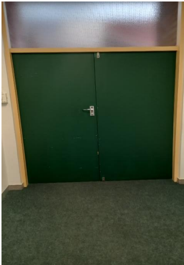
Existing door and frame to be painted
