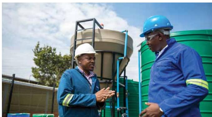
◀ Left: The mine wastewater pilot plant currently takes about eight hours to treat 3 500 L. Recoveries can be increased by increasing the size of the plant. The plant can also be packaged in a modular form or can be semi-mobile, depending on end-user requirements. ▲ Above: CSIR chemical engineer Rhlulani Shingwenyama (left) is responsible for the design, sizing and construction of the plant.
