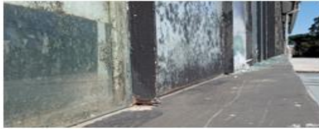
Photo 2.5: Bottom window sill with glazing fixed to steel frame (rust visible) with silicone visible behind it. Broken glass pieces also visible further down.
