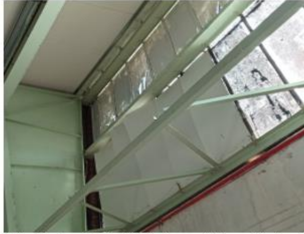
Photo 2.8: Inside view of glazing that has been painted over. Hardboard covers had also been placed over some of the elements and some of these boards have broken and become loose. The wind girder at the low level can possibly be used to build an access platform on, for working on the glazing from the inside.
