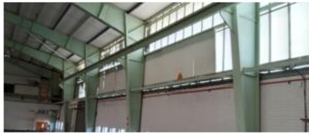
Photo 2.9: Glazing elements on South Façade with timber boarding at some of the window panels.
