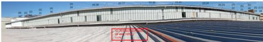
Photo 2.11: North Façade with number of cracked glass panels noted above each of the structural bay numbers.
