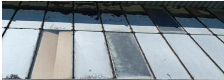
Photo 2.3: Glazing with steel frames with varying glazing elements ( +/- 2.1m x 0.6m in size). Each glass panel weighs about 20kg.
