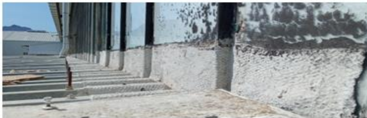
Photo 2.4 : Low level roofs have waterproofing onto the existing glazing. Removal of these glazing elements will require re-waterproofing which will be additional costs to the project.
