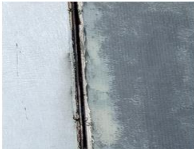
Photo 2.7: Glass frames with visible fibres coming off from the glazing.
