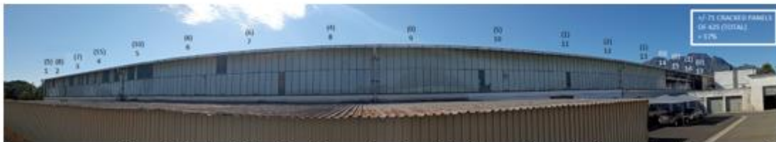
Photo 2.10: South Façade with number of cracked glass panels noted above each of the structural bay numbers.
