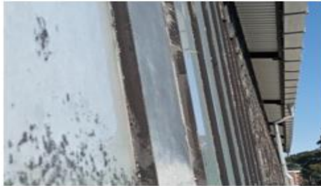
Photo 2.6: Glass frames with visible fibres coming off from the glazing. Samples were sent off for analysis. See attached Annexure A report from Beam Analytical, related to asbestos fibre testing, that had a positive result.
