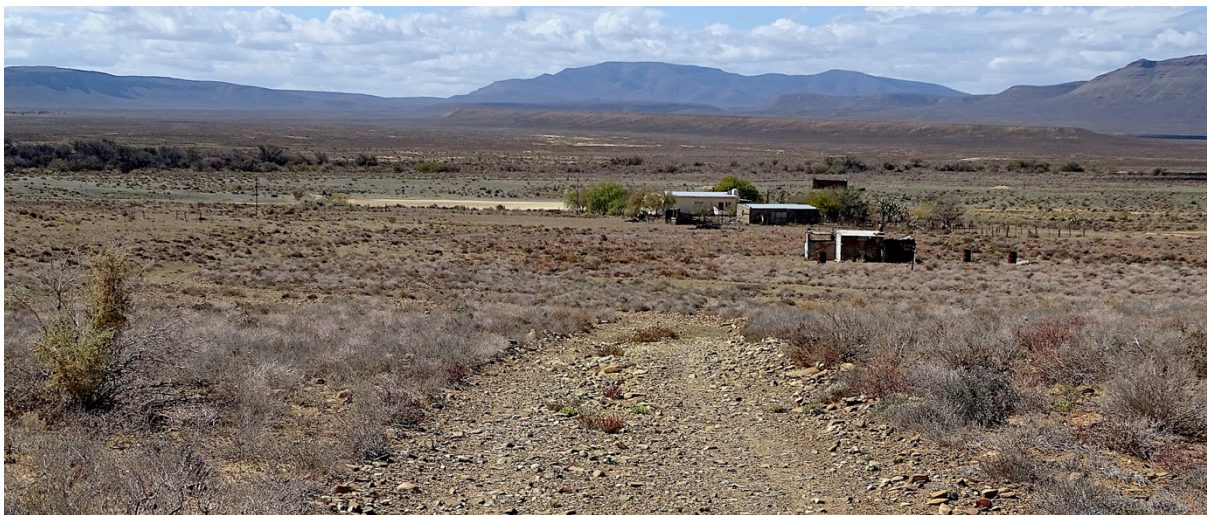
Figure 2: Grootfontein homestead in river plain, looking north-east
