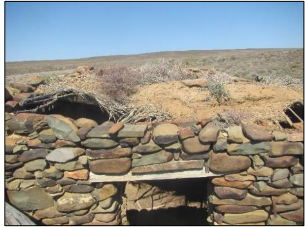
Figure 32: Roof detail of the ruin at waypoint 158 showing the brakdak.
