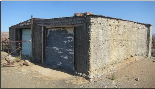
Figure 41: Outbuilding at waypoint 201 showing a combination of traditional and modern materials.
