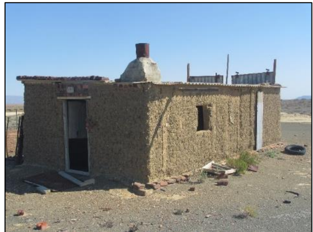
Figure 44: Cottage at waypoint 203 showing a combination of traditional and modern materials.
