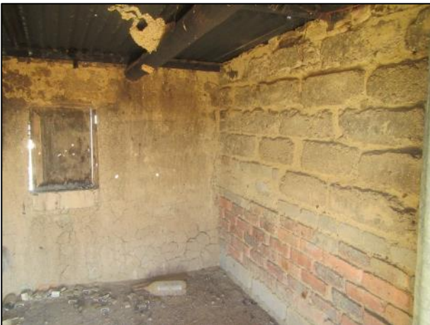
Figure 43: Interior of the labourer's cottage at waypoint 202 showing construction materials.
