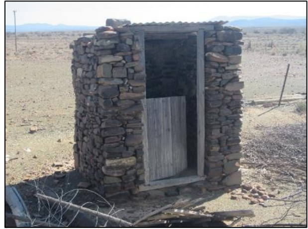
Figure 40: View of the outside toilet at waypoint 201.
