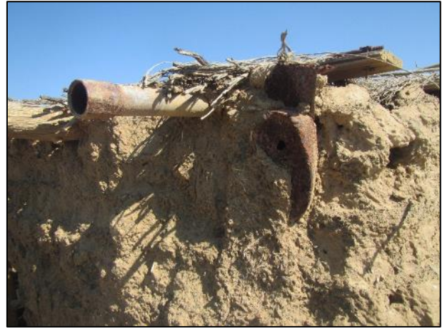
Figure 24: Detail showing the use of metal in the roof structure.
