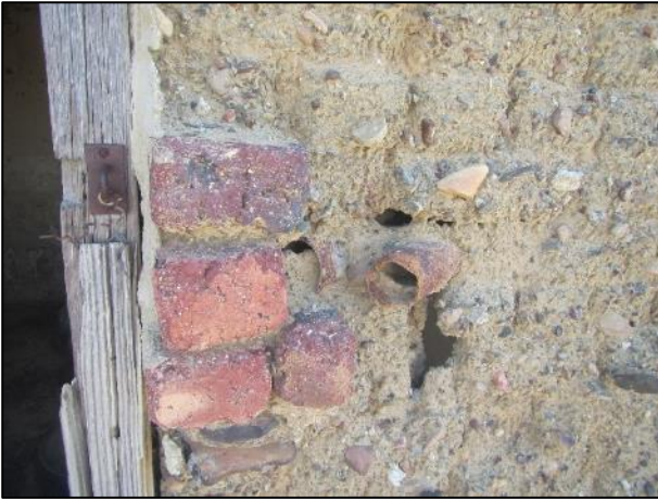
Figure 45: Detail of door frame and metal pipes supporting the internal hearth inside the cottage at waypoint 203.
