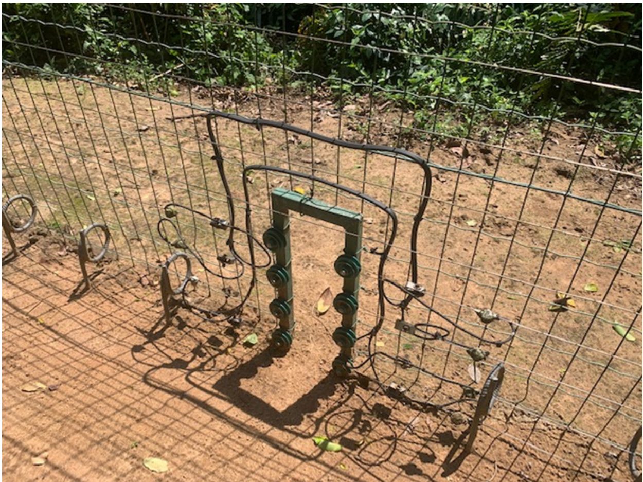
Figure 28. Image showing “critter path” within electrified fence. Similar measures should be implemented on the site.
