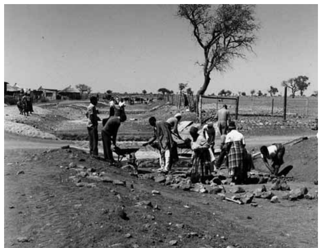
Figure 6.19: Roadside drains of the major system
