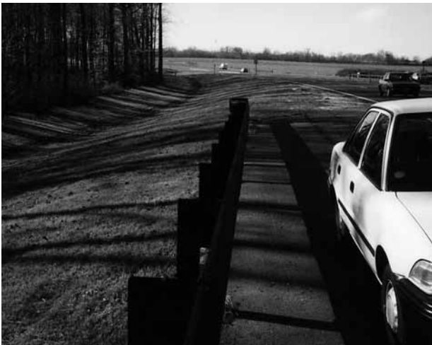
Figure 6.16: Open channel alongside an arterial road
