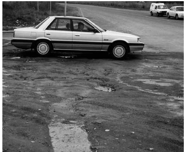
Figure 6.14: Flow across this intersection has resulted in siltation, which is inconvenient and hazardous to road users
