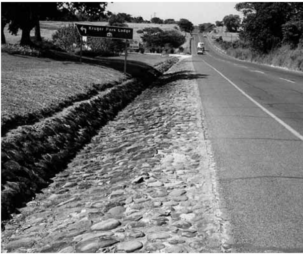
Figure 6.11: A lined open roadside channel
