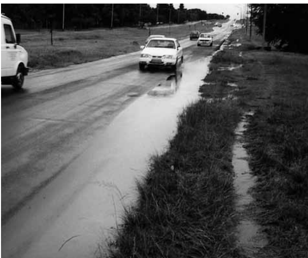
Figure 6.13: This ponding is the result of encroachment of the grass verge onto the road. Grass-cutting maintenance operations should also include harvesting the grass, to prevent siltation and build-up of new grass growth
