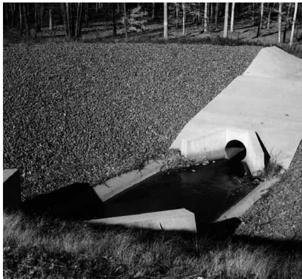
Figure 6.7: Multiple-outlet structure of a detention pond
