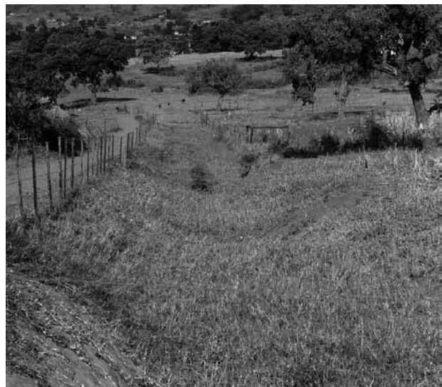
Figure 6.24: An example of a grassed waterway
