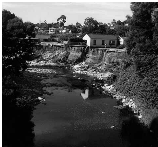
Figure 6.2: Damage from major floods can be catastrophic
