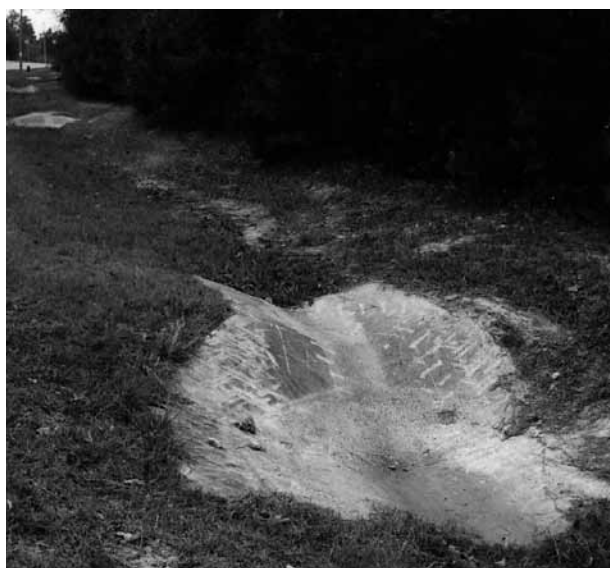
Figure 6.8: Simple drop structures in a residential environment
