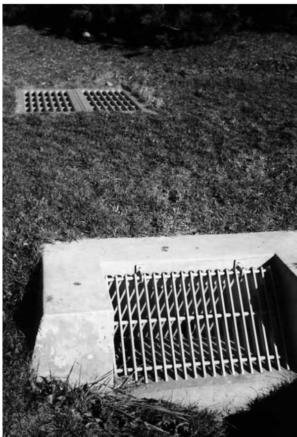
Figure 6.22 (a): Depressed area to store excess runoff
