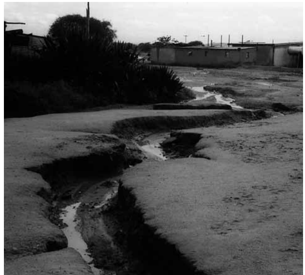
Figure 6.18 (b): Concentration of stormwater drainage in a roadway resulting in major inconvenience to road users
