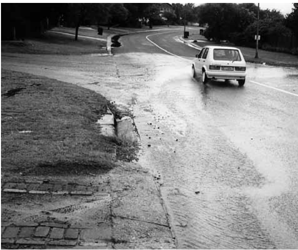
Figure 6.12: Incorrect vertical alignment has caused stormwater to bypass this kerb inlet. Kerb inlets in the intersecting road on the left have also not captured runoff from that road so that stormwater flows across this bus route, creating a hazard
