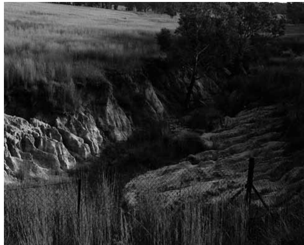
Figure 6.23: Gully erosion by headwater upstream of a highway culvert inlet. Specific attention needs to be paid to structures founded in soils with high erosion potential
