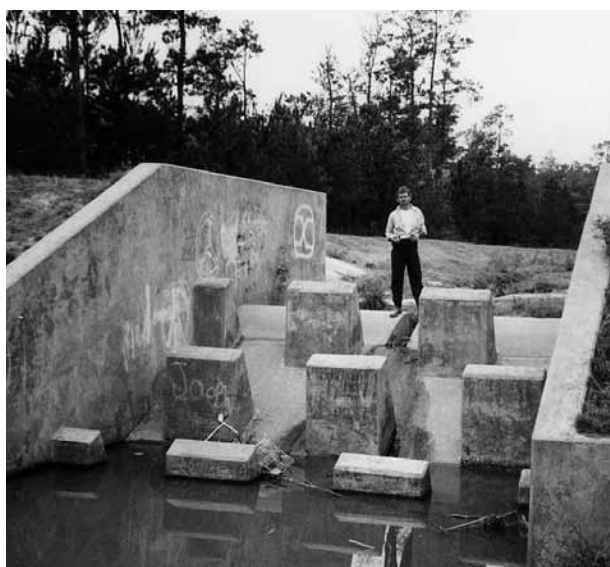
Figure 6.9: Energy dissipator
