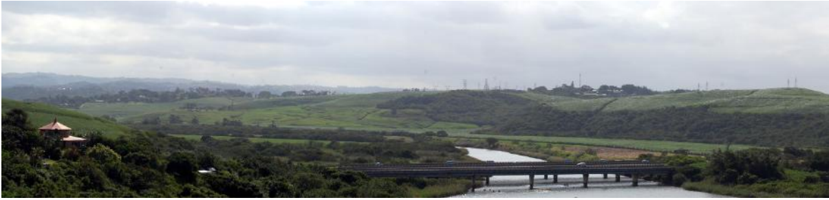
Figure 10-48 View north-west from LVP017, northern Illovo Beach, across the Lovu River floodplain. The Kingsburgh Major Substation is visible on the hills in the middle, as are the N2 and R102 bridges across the river.
