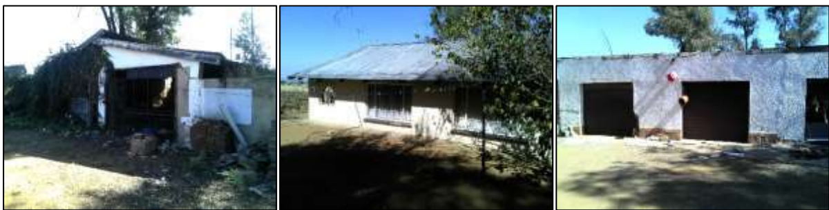
Figures 17 & 18: Two other residential buildings.
