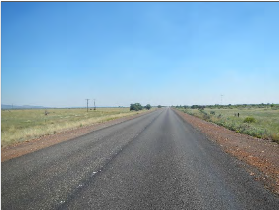
Figure 14: Typical view of the R31 main road
