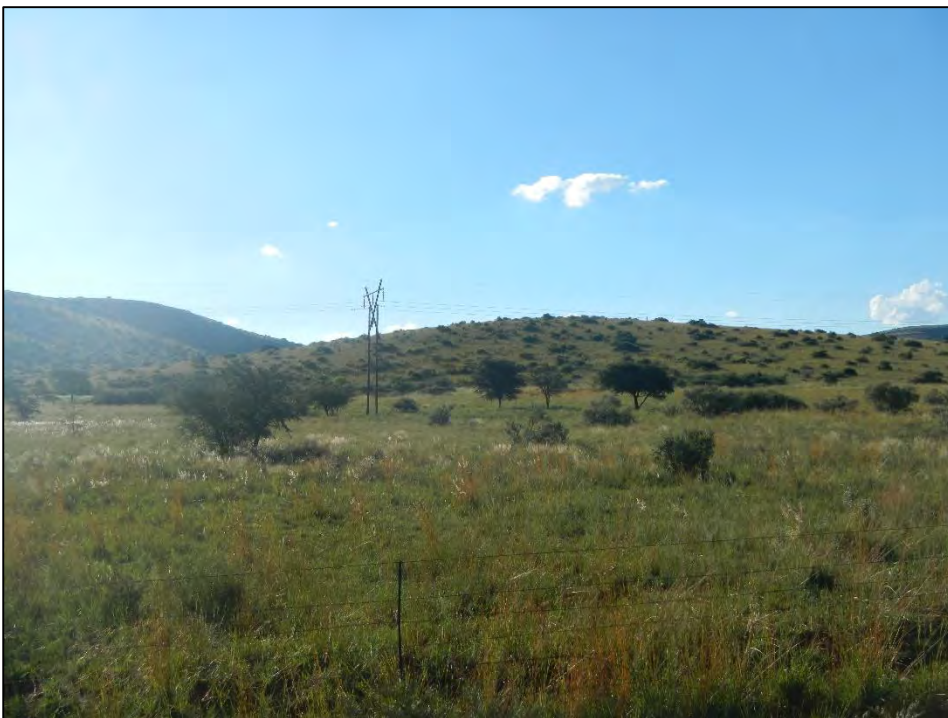
Figure 12: Typical view of the existing medium voltage power lines which can be found within parts of the study area
