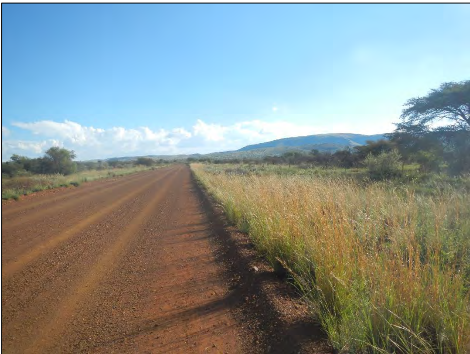
Figure 10: Typical view of the gravel access roads which can be found within the study area
