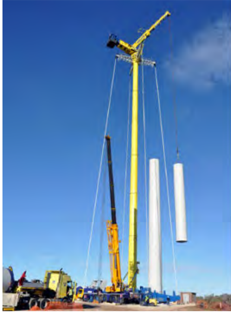
Figure 14: Cranes at work
