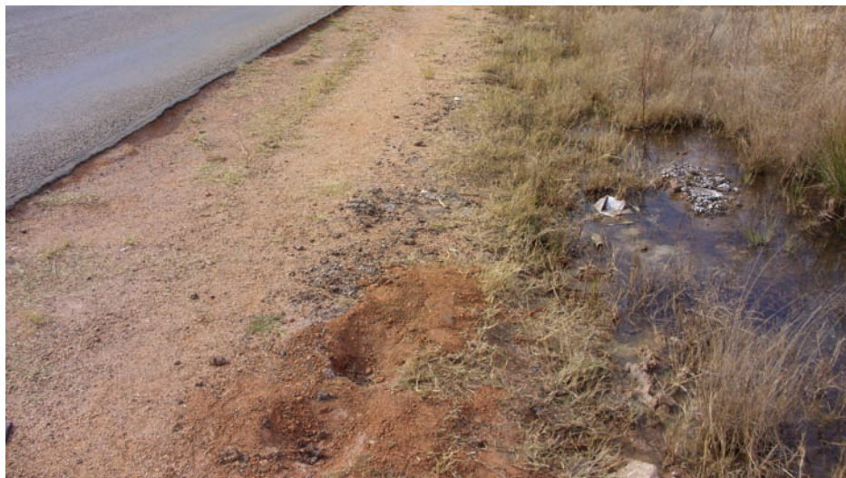
Figure 1: Localised ponding of water from seepage in the adjacent area during the dry season (note the presence of hydrophilic plants near the road)
