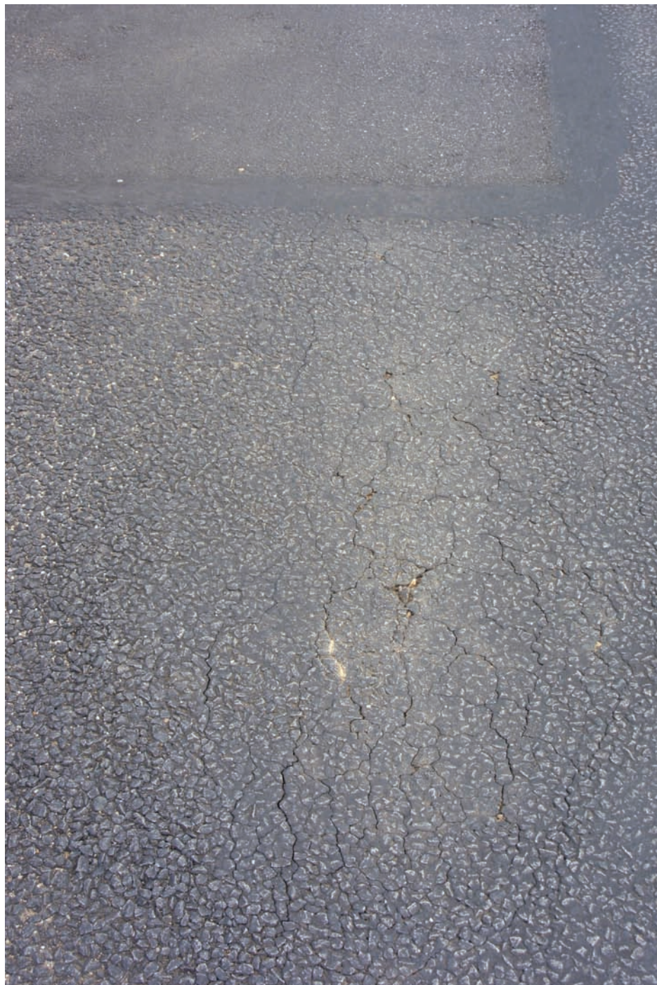
Figure 12: Fatigue cracking of a thin bituminous seal with pothole formation
