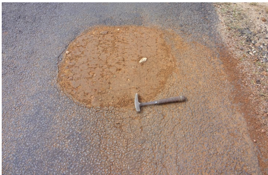
Figure 13: A pothole (filled with roadside material) resulting from unsealed cracks in a thin bituminous surfacing
