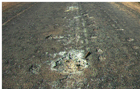
Figure 16: A pothole developing as a result of excessive soluble salts in the pavement base layer
