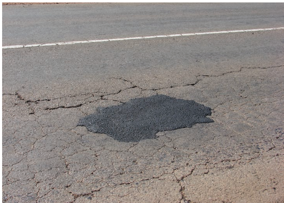
Figure 30: A poorly-finished and untidy patch
