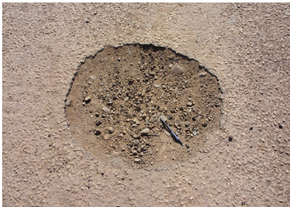
Figure 8: A typical pothole formed under a thin surfacing with a granular base
