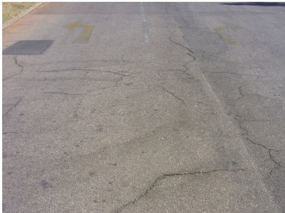
Figure 3: Cracking of asphalt resulting from ageing
