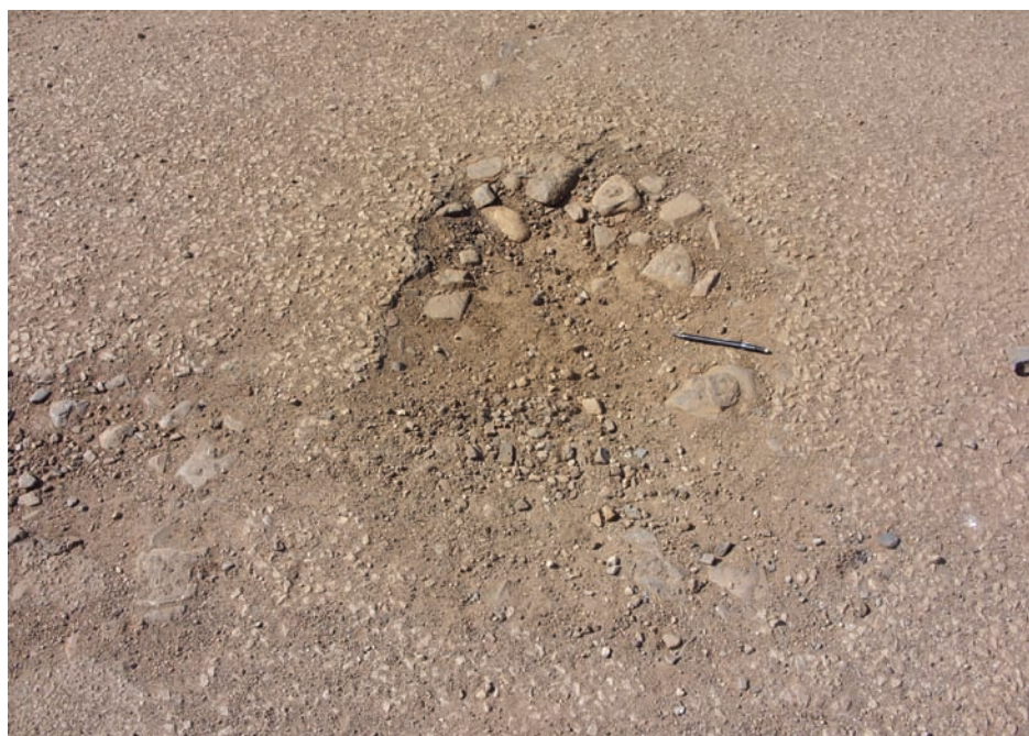
Figure 9: A pothole resulting from large stones in the base beneath the seal
