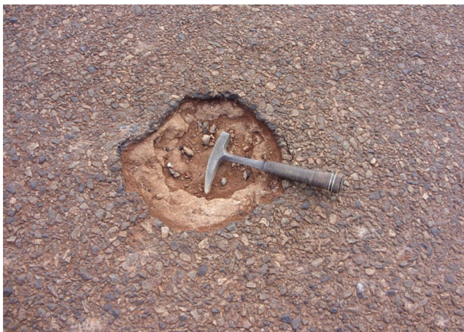
Figure 11: A pothole resulting from lamination, carbonation and weak layers in the top of a stabilised base material
