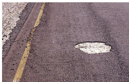
Figure 14: A typical pothole formed as a result of carbonation of a stabilised base
