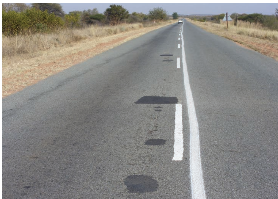
Figure 25: Potholes resulting from construction deficiencies
