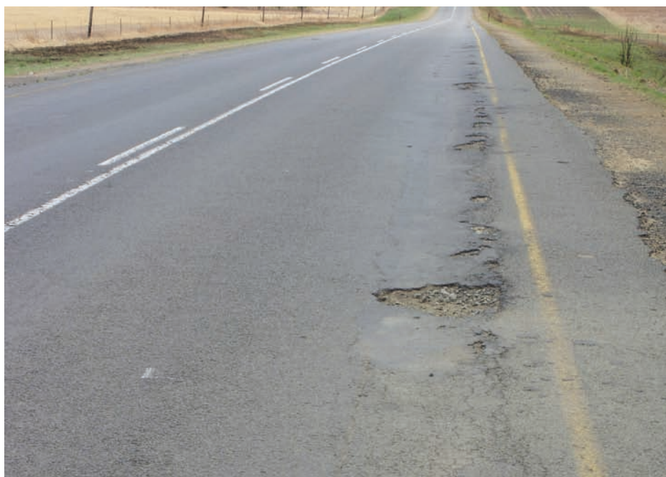
Figure 26: Long, linear development of potholes, resulting from inappropriate layer materials
