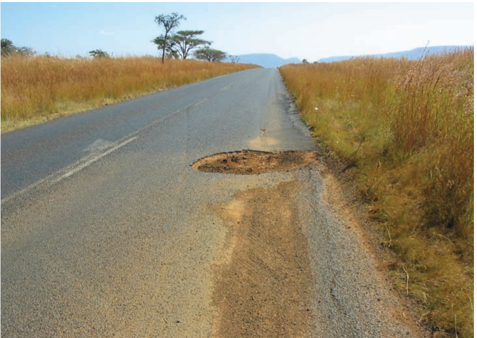
Figure 23: Enlargement of an unrepaired pothole through ravelling and whip-off
