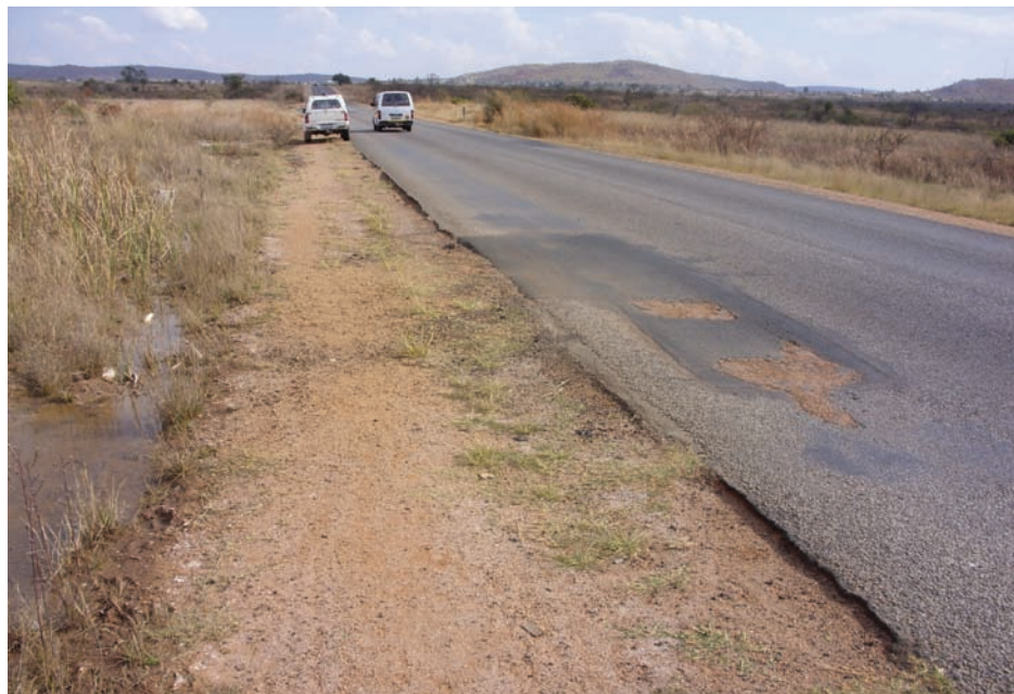
Figure 19: Failure of a patch within one year of repair – note standing water adjacent to the road in this area
