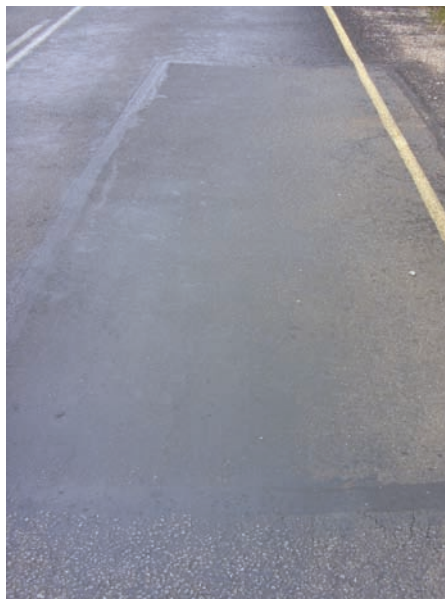
Figure 28: The effective use of a geosynthetic crack-sealing strip to seal the edges of a patch
