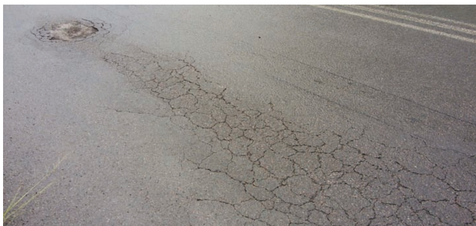
Figure 2: Typical fatigue-cracking of asphalt leading to a pothole
