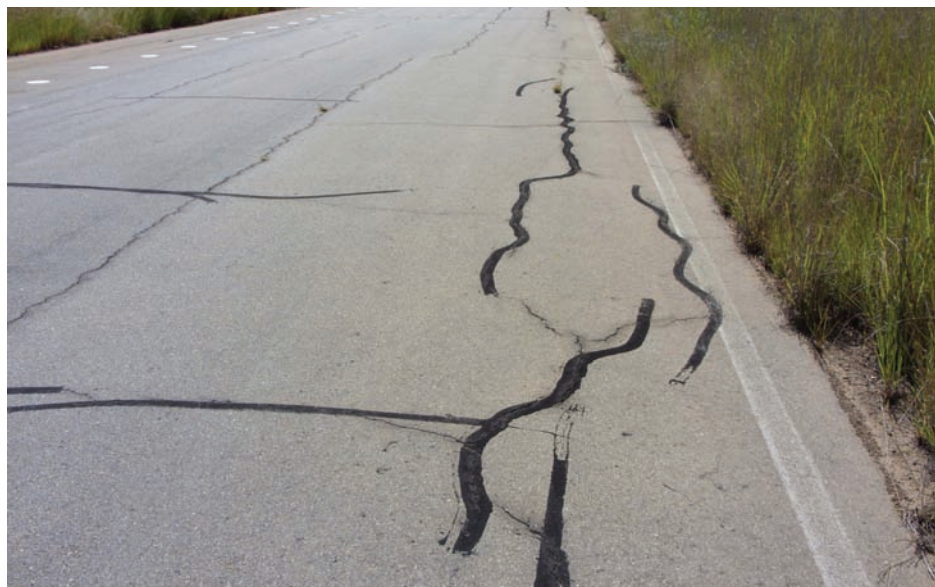
Figure 4: Typical reflection-cracking of stabilised material through a G1 base and 30 mm of asphalt (mostly sealed)
