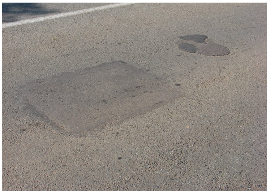
Figure 31: A well-executed and aesthetically-pleasing rectangular patch next to a less effective 'circular' patch
