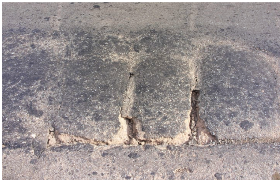
Figure 6: Initiation of potholes as a result of overloading of a stabilised base – initial cracking followed by pumping and then potholes
