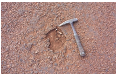
Figure 15: The initiation of potholes due to a lack of prime
