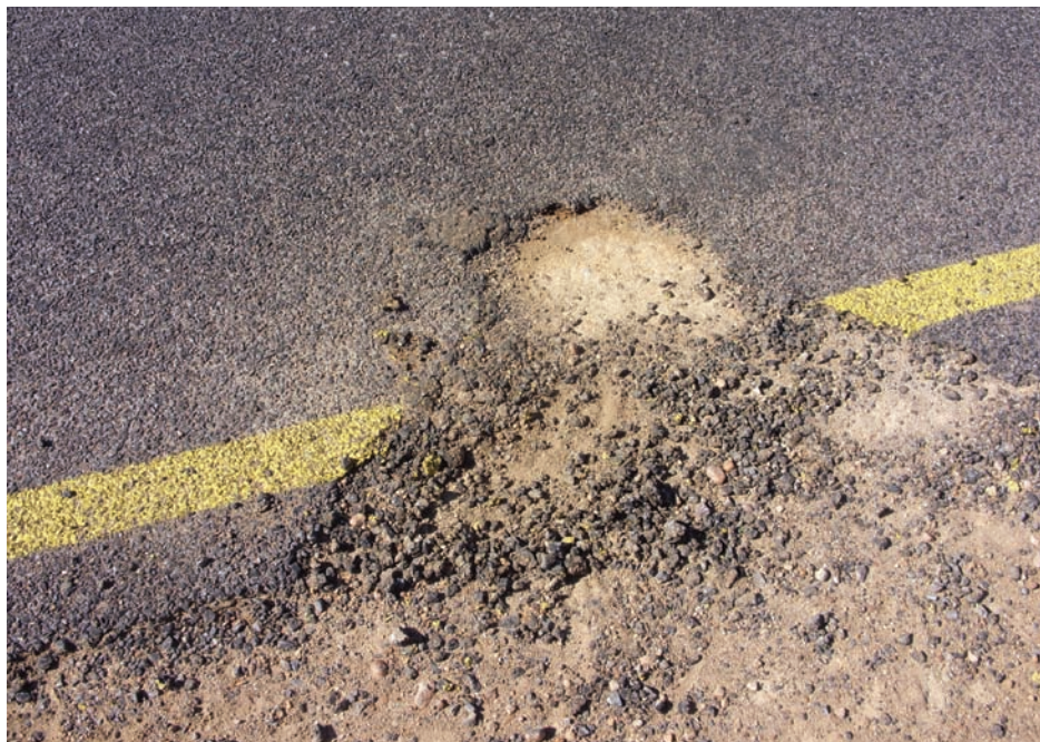
Figure 10: A typical pothole resulting from a weak upper-layer of stabilised material
