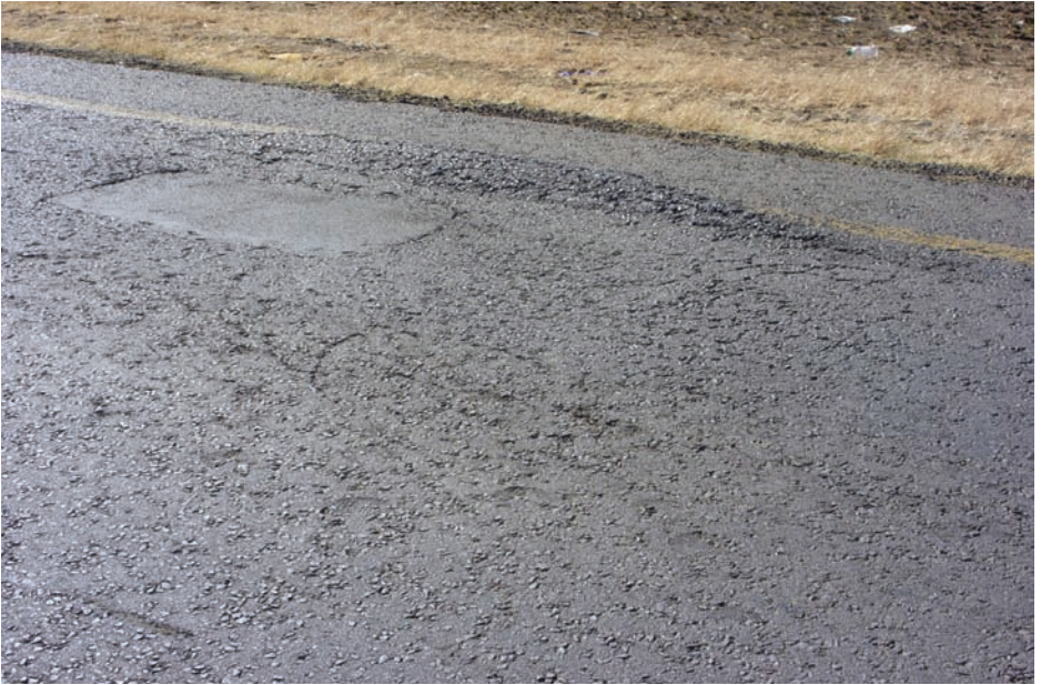
Figure 22: Shear failure in the base (note heaving of the asphalt adjacent to the yellow line) and a patched pothole that formed
