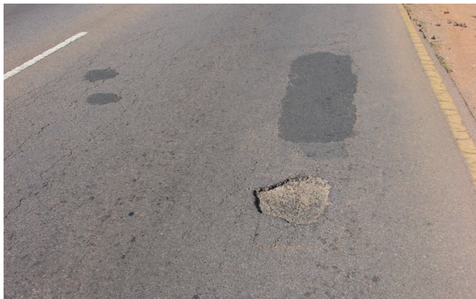
Figure 5: Typical shallow failure of asphalt at the interface with older asphalt
