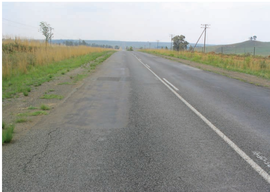
Figure 24: Moisture/traffic-associated cracking in the outer wheel track leading to potholing and extensive patching
