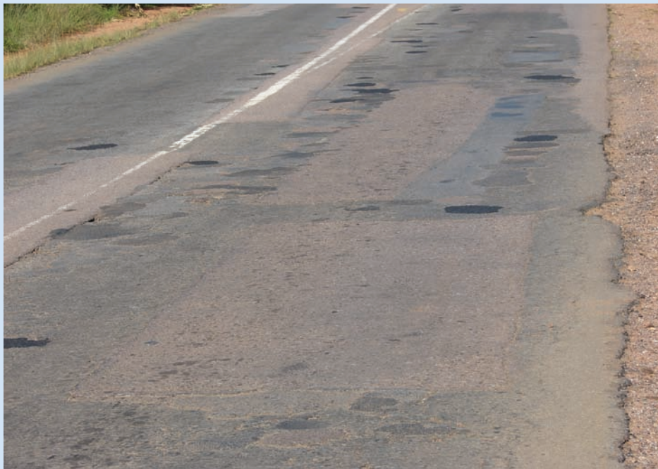
Figure 27: Repeated repair of potholes due to the fundamental problem (subsurface drainage) not being addressed
