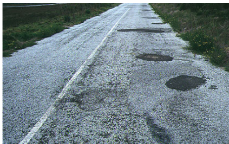
Figure 17: Repaired potholes caused by mole-rats
