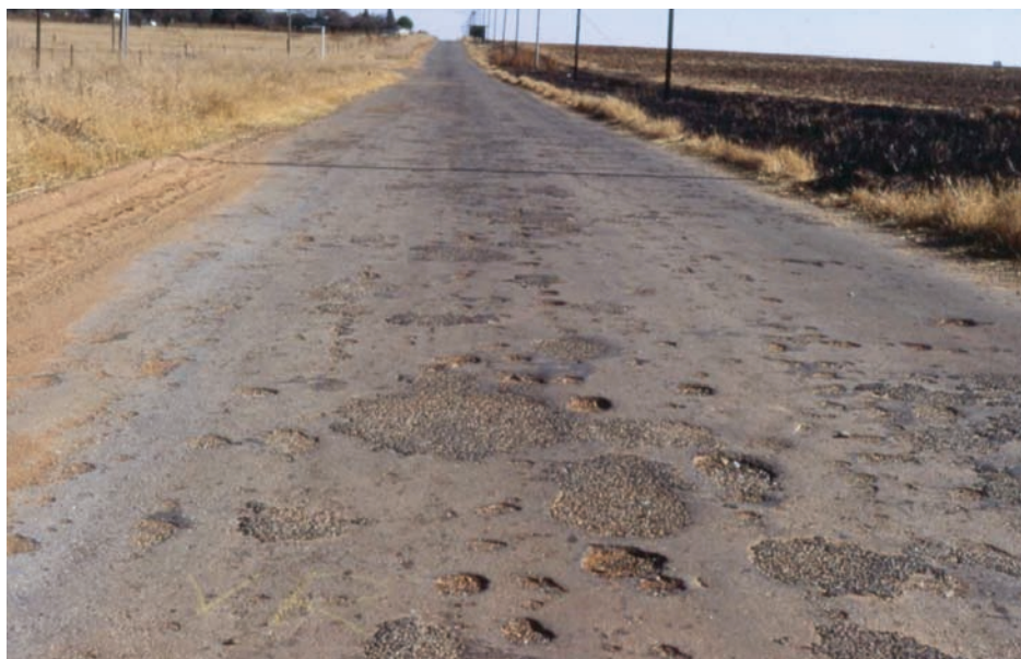
Figure 7: Development of potholes on a low-volume road with thin bituminous surfacing and insufficient preventative maintenance
