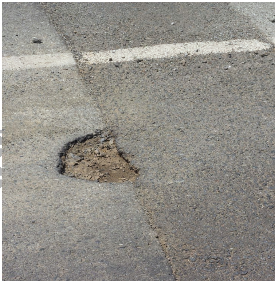
Figure 18: A typical pothole formed adjacent to a service trench
