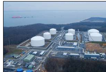
Dominion Cove Point LNG terminal with a capacity of 0.4 bcm storage (LNG); 18.6 bcm/a regasification
