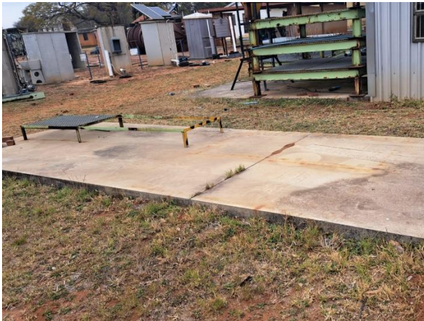
Figure 16: Concrete Slab for Demolition – 3.0mx20m
