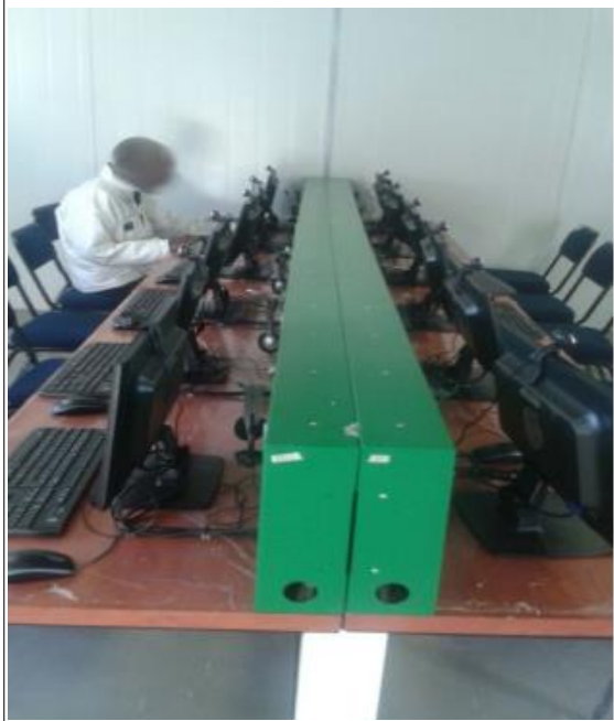
Figure 3: Lip Channel ICT Centre Installation
