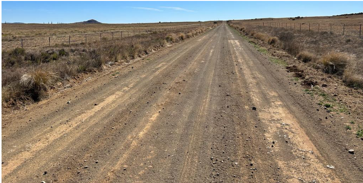
Figure 2.8: Photo of the S1262 taken along the gravel portion of the road (Source: Sturgeon Consulting, 2023).
