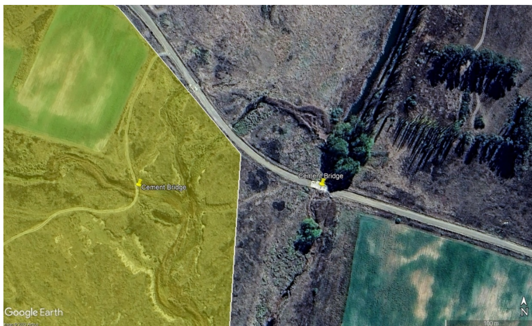
Figure 2.4: Map indicating the relevant cement bridges (Source: Google Earth, 2023).
