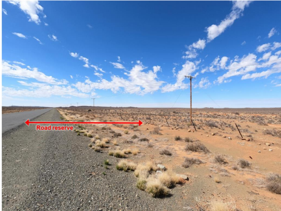
Figure 31: Typical characteristics of the road reserve in the proposed Fibre Optic Project study area. The road reserve varies in width, and can be very narrow some places. Photo: L. Snyman-van der Walt, site visit, 17 November 2021.
