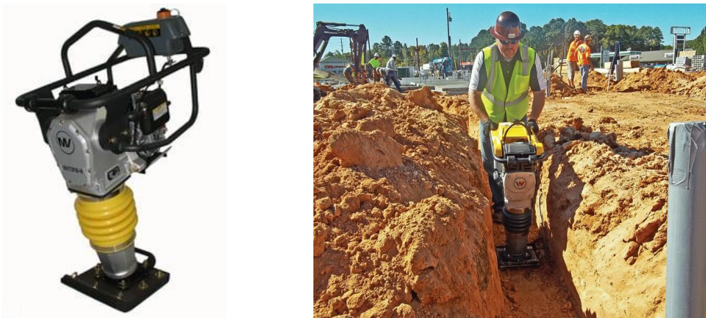
Figure 3: Example of trench backfilling and compaction.
