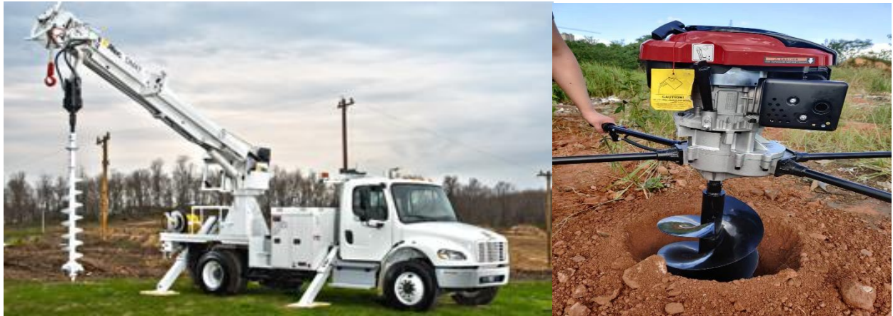
Figure 7: Holes for installing overhead cabling poles will be dug by truck-mounted (left) or hand-held (right) drills.
