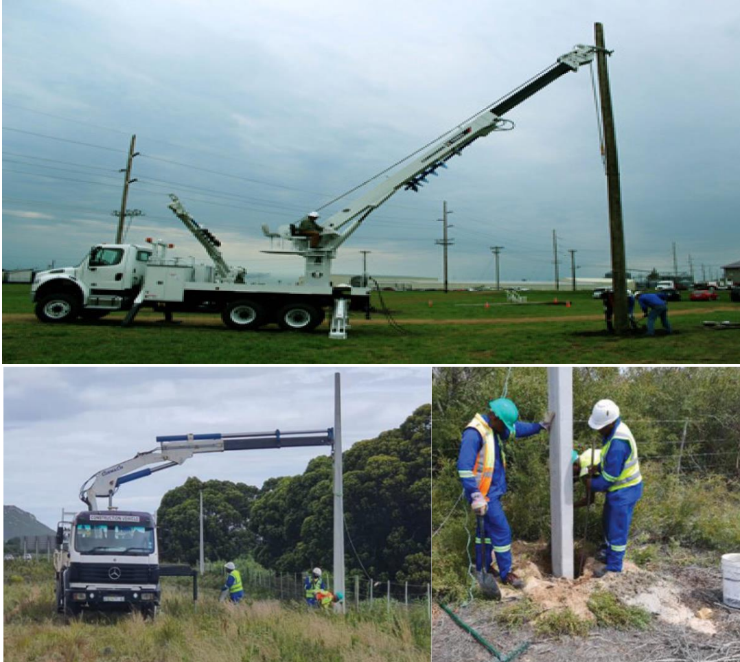
Figure 9: Example of a truck used to plant timber (top) and concrete (bottom) poles.
