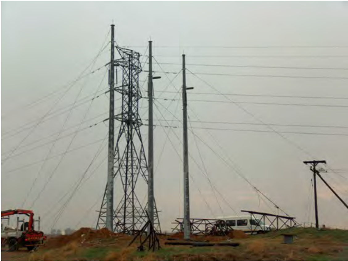
Figure 1-23 An example of monopole towers next to a lattice type tower for 132 kV power lines. (Source: http://www.rame.co.za/flagship-projects/132kv-lattice-to-mono-pole-replacement/nggallery/image/578 )
