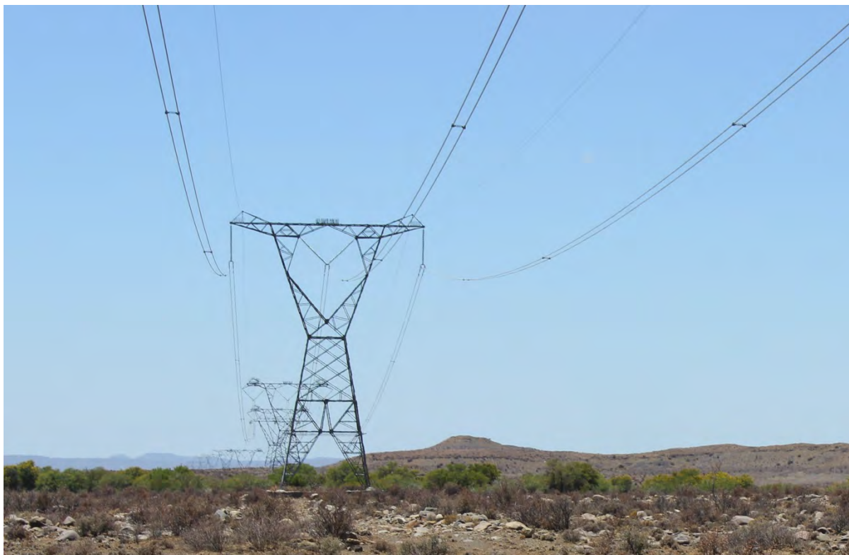
Figure 1-21 High voltage power lines crossing the road at SVP025 (looking east).
