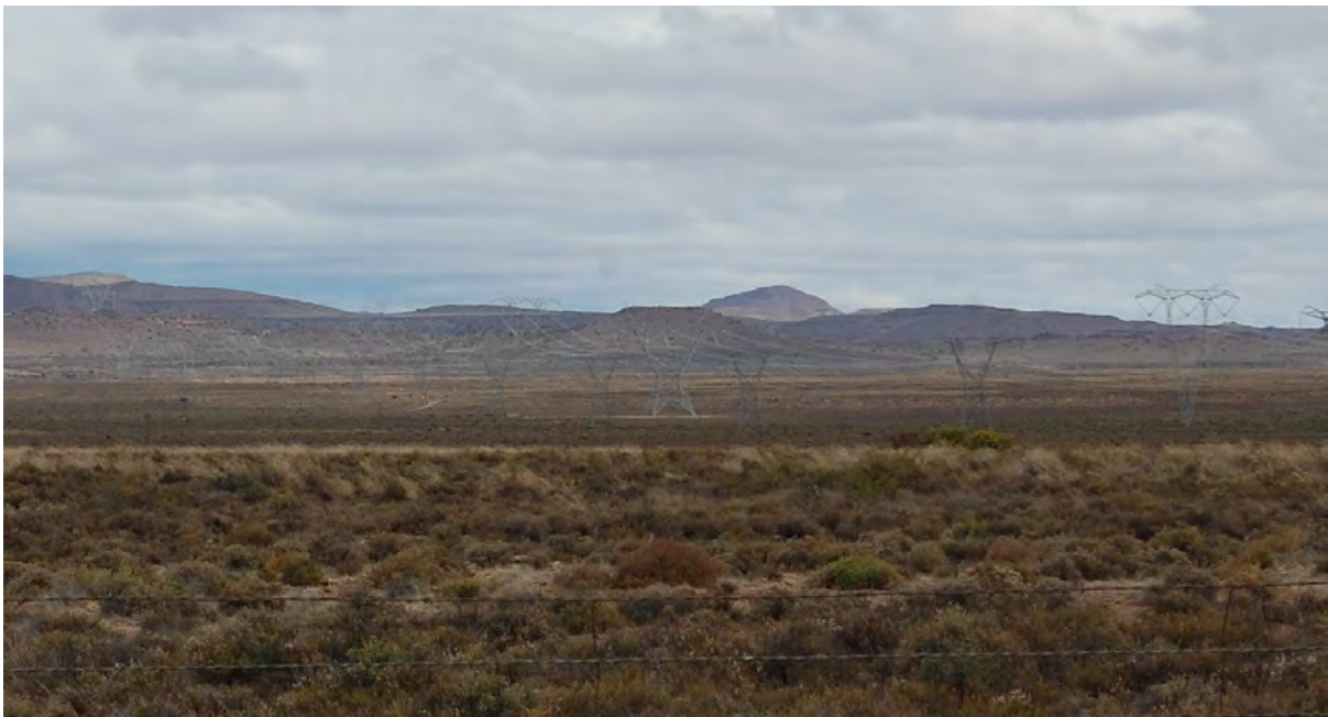
Figure 1-24 High voltage transmission lines with lattice towers against a mottled landscape similar to that of the Sutherland region (photo taken by author).
