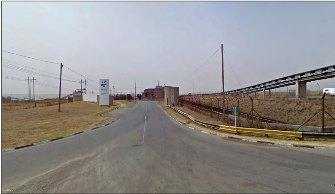
Figure 3-49: Substation and coal conveyor adjacent to the Riaan Rademan Training Academy (Source: Google Earth 2022)
