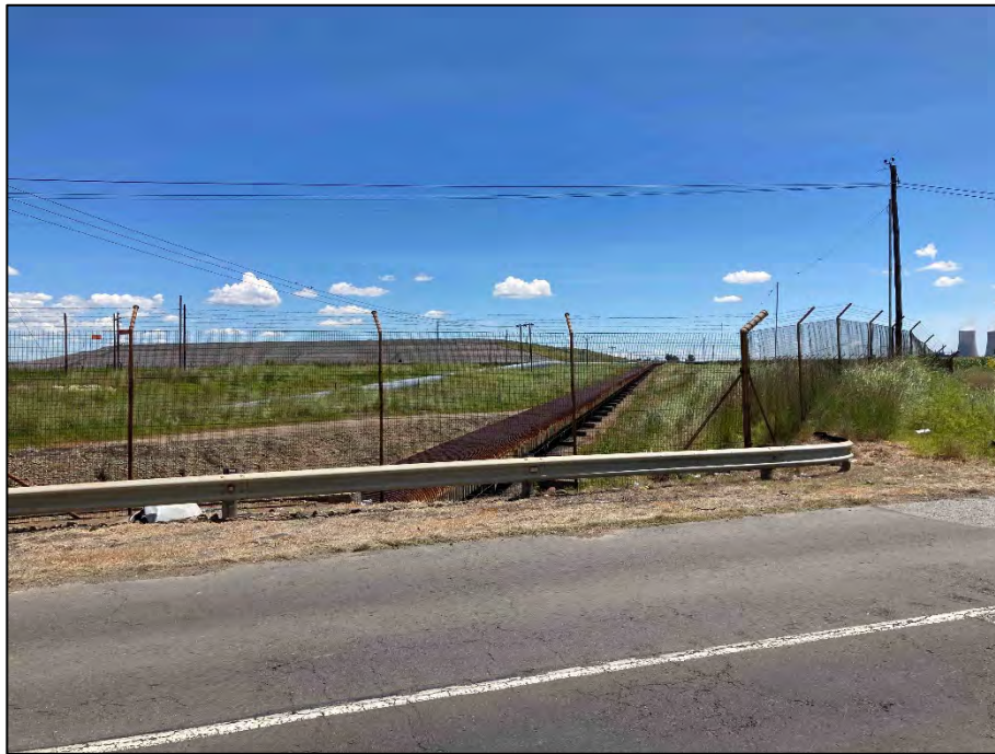
Figure 3-47: Infrastructure associated with the Sasol Plant
