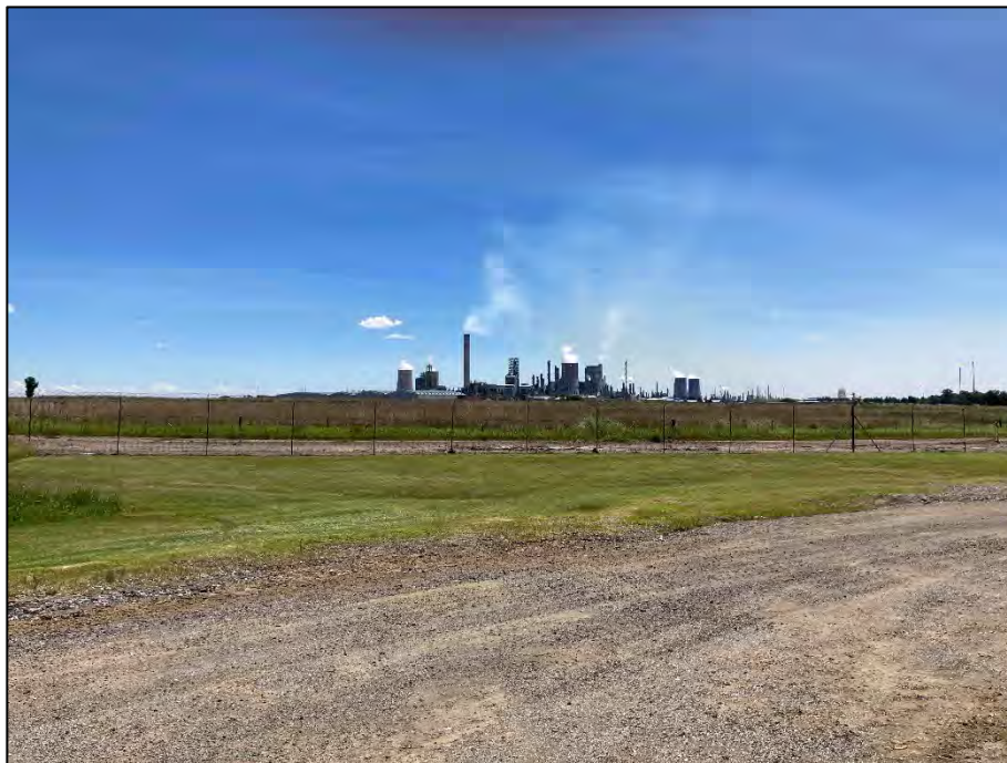
Figure 3-46: Sasol synthetic fuel plant located on the western boundary of the Vhuvhili SEF study area.
