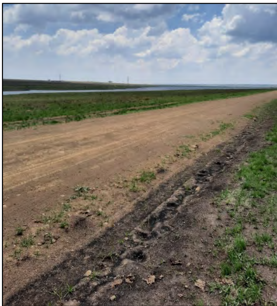
Figure 3-58: Gravel road with a dam in the background.
