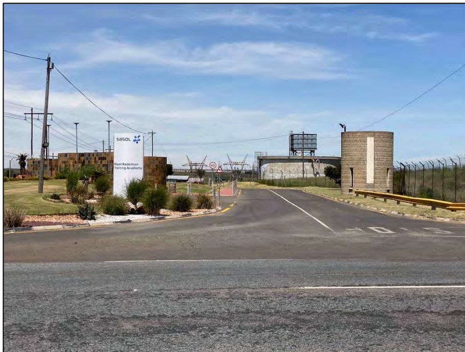
Figure 3-48: Riaan Rademan Training Academy located close to the Sasol Fuel Plant
