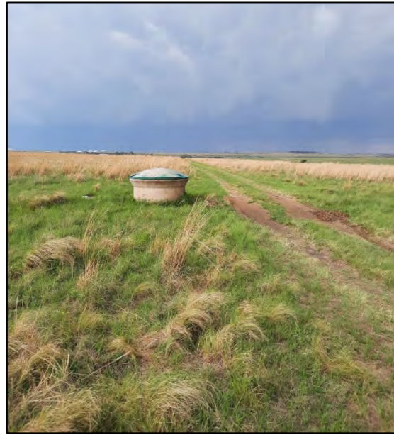
Figure 3-57: Grass cover and a pipeline manhole.
