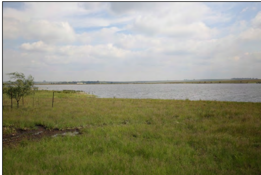
Figure 3-18: The main dam on the proposed Vhuvhili SEF site.
