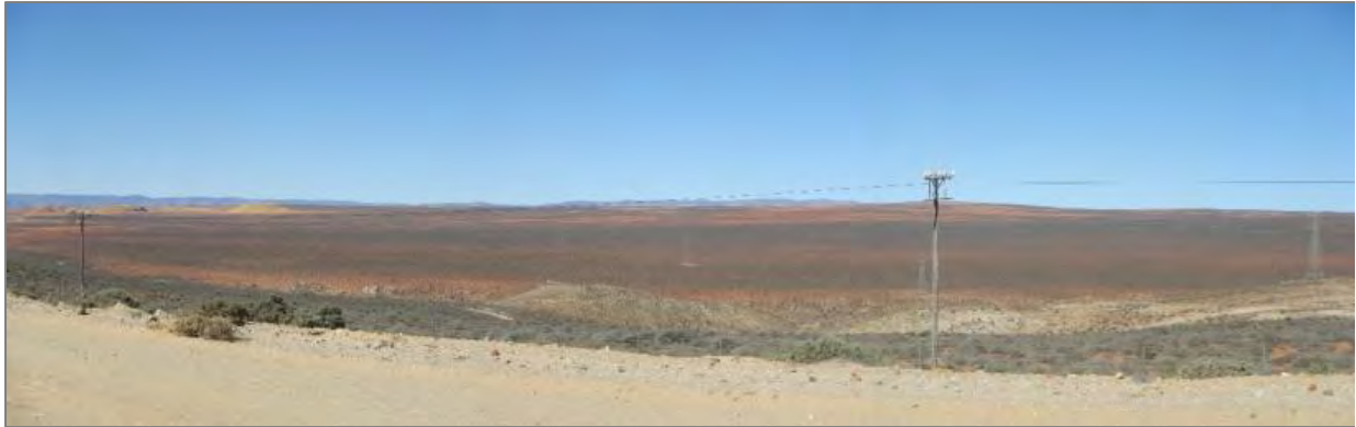
Figure B8.6. View towards the south from the vicinity of the Gromis Substation. The mining on Mannels Vley is visible at the far left.
