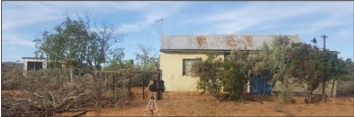
Figure B8.11. View of the front of the Kapvlei farmhouse. The overall form and the presence of steel-framed windows are typical of early-mid-20 th century structures in the region. Photo provided by Morné de Jager.
