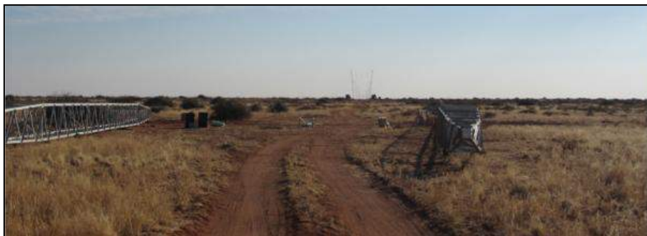
Figure 8: View northwards along the western margin of the site showing a new power line currently under construction.
