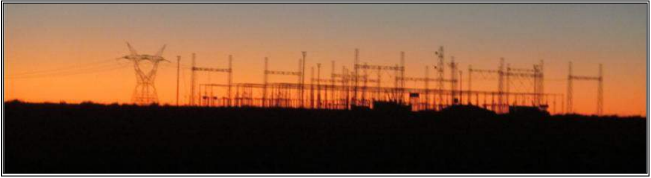
Figure 24: Evening view of the large Eskom substation located some 16 km south of the proposed project.
